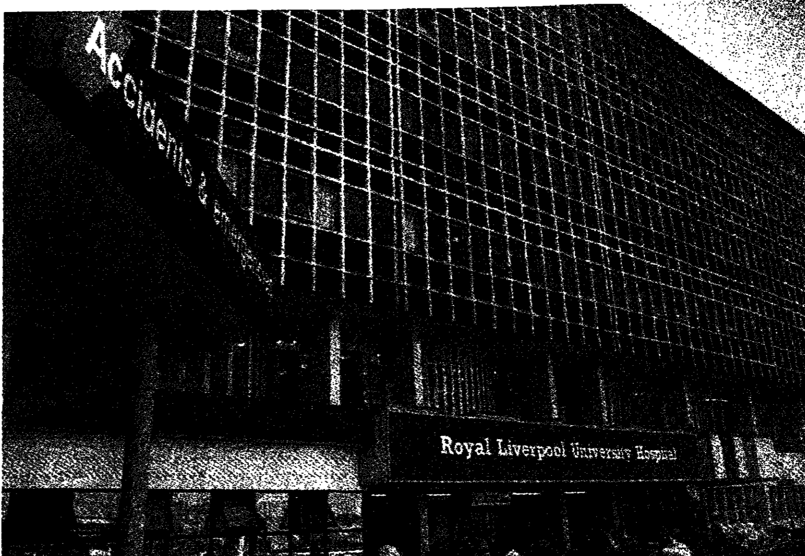
A Liverpool hospital where facilities management has been contracted out to Mowlem. Will the industry, in the future, polarise into services and management companies?
